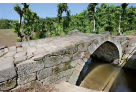
Bridge of Veiga (Lousada). Upstream view.
