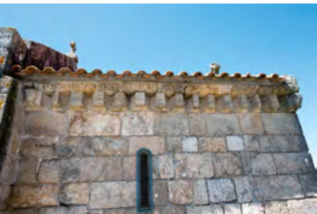
Chapel of Quintã (Paredes). South façade. Chancel.
