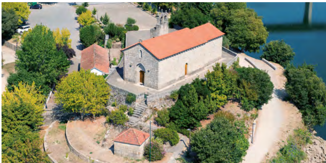
Church of Sobretâmega (Marco de Canaveses). Aerial view.
