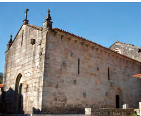
Monastery of Ermelo (Arcos de Valdevez). West and south façades.
