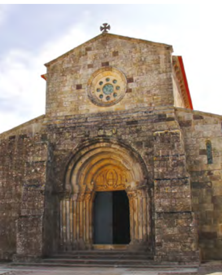
Church of São Pedro de Rates (Póvoa de Varzim). West façade.
