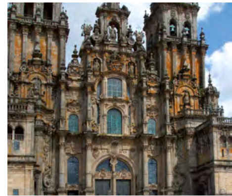
Cathedral of Santiago de Compostela (Spain). West façade. Partial view.
