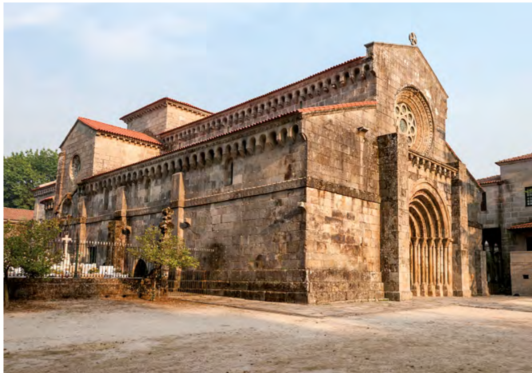
Monastery of Paço de Sousa (Penafiel). General view.
