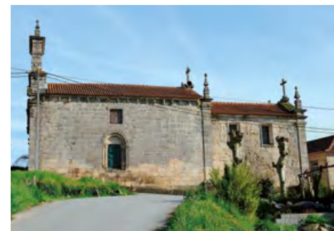
Church of Veade (Celorico de Basto). North façade.
