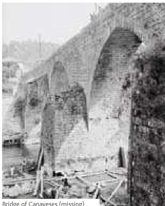
Bridge of Canaveses (missing)
