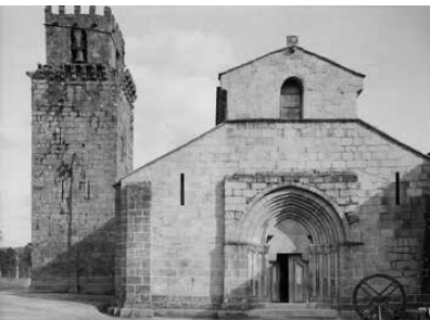
Church. West façade before the intervention carried out by the DGEMN. Source: IHRU archive.
