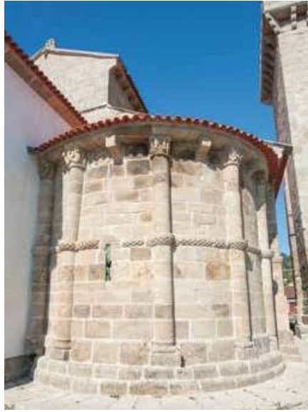
Church. North apse chapel.
