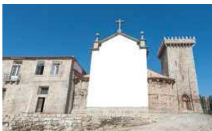
Church. East façade.
