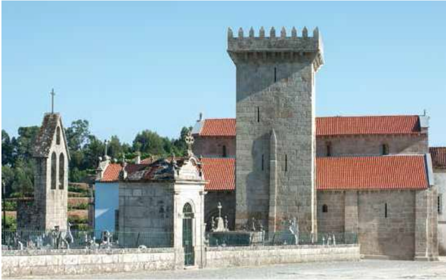
Church and tower. North façade.
