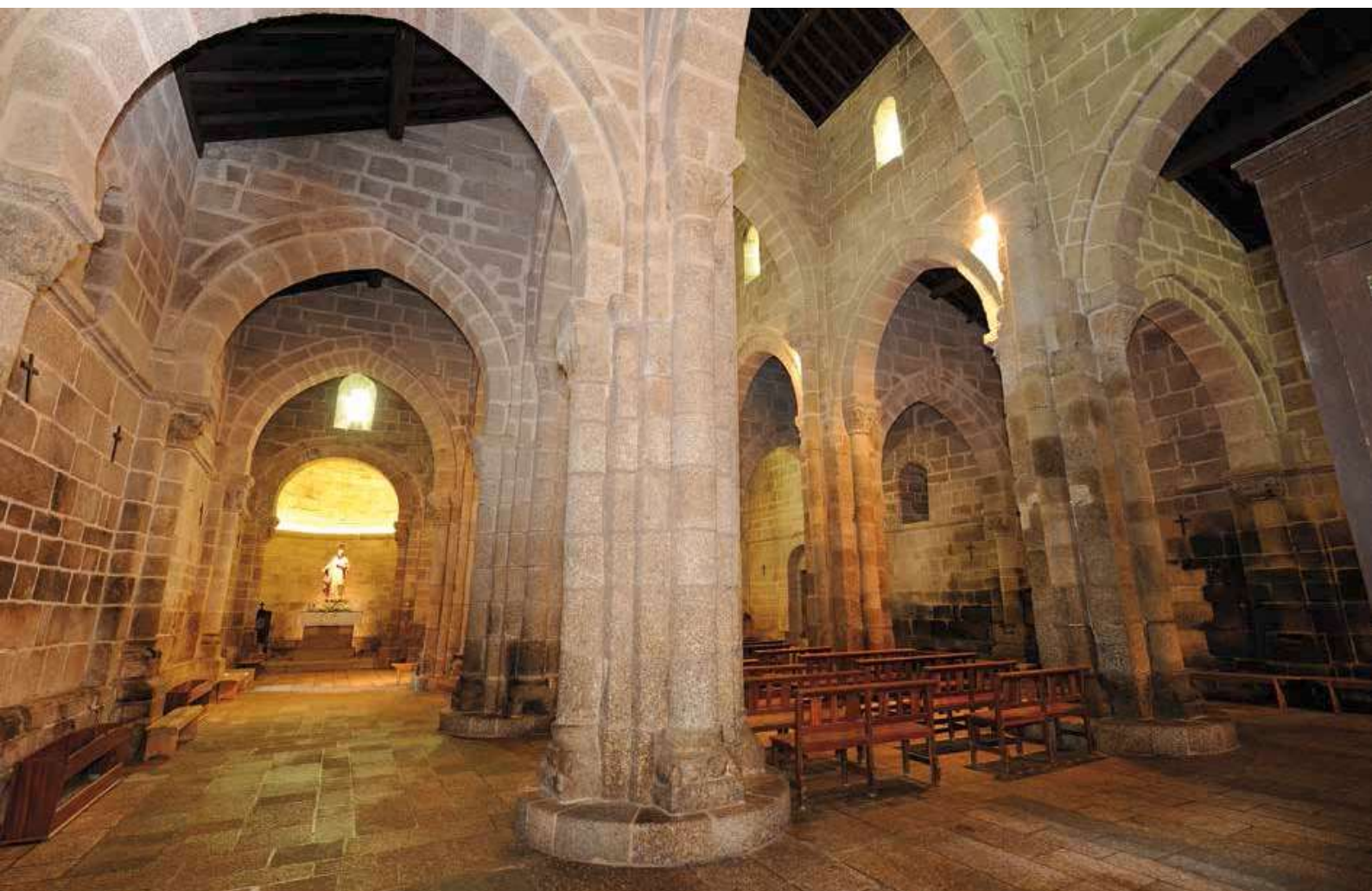
Church. Naves. Diaphragm arches.
