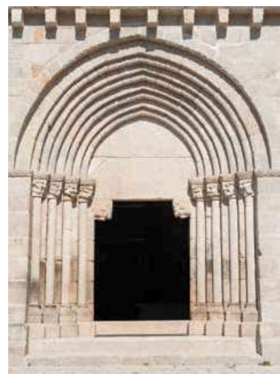
Church. West façade. Portal.
