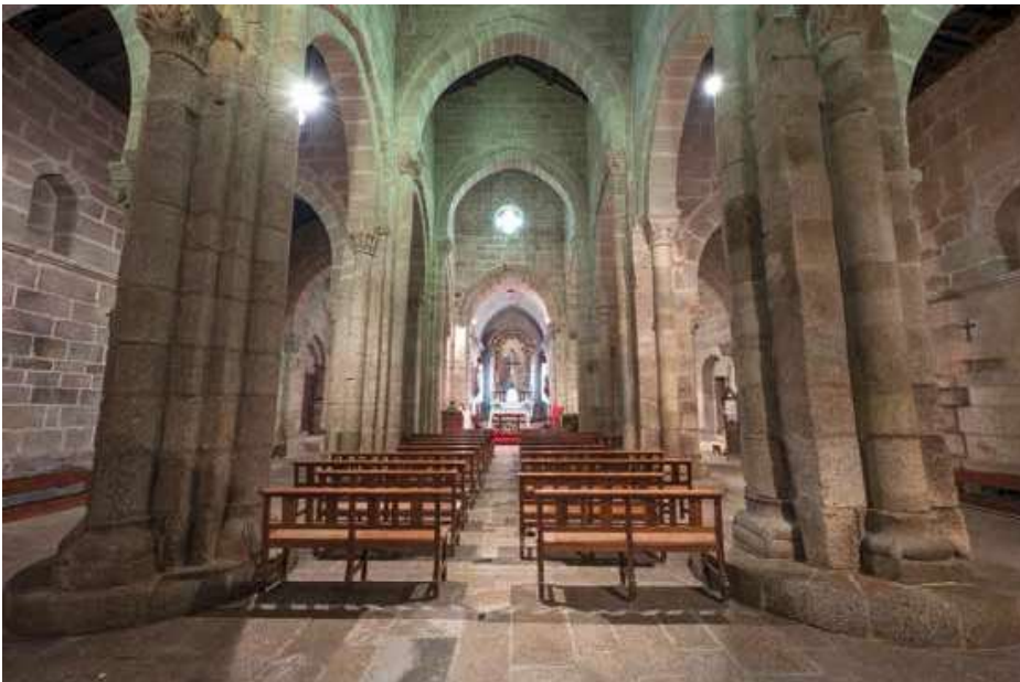
Church. General interior view from the central nave.
