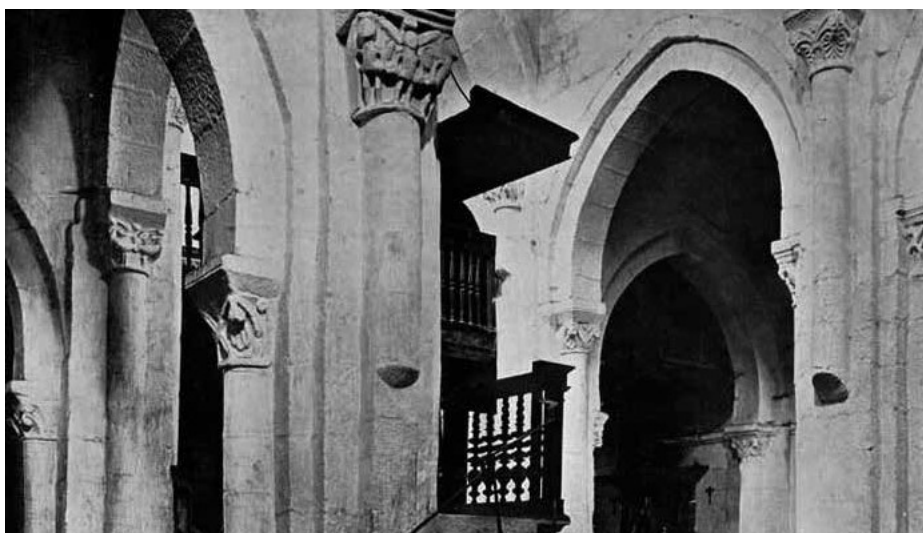
Church. Interior view before the intervention carried out by the DGEMN. Source: DGEMN's Bulletin no. 15.
