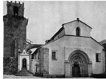
Church. West façade and tower before the intervention carried out by the DGEMN. Source: DGEMN’s Bulletin no. 15.
