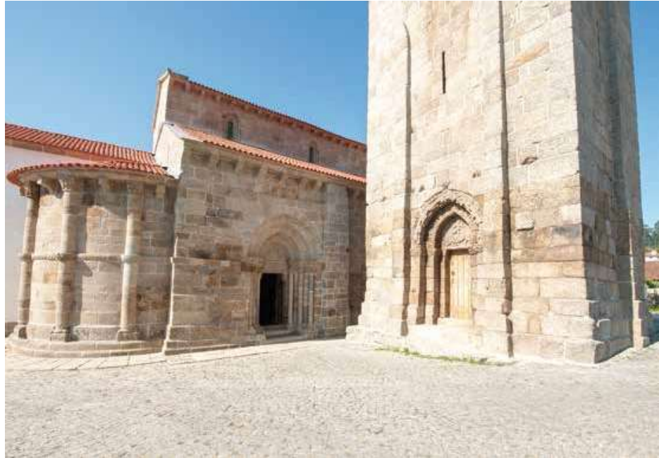
Church. North façade and tower.
