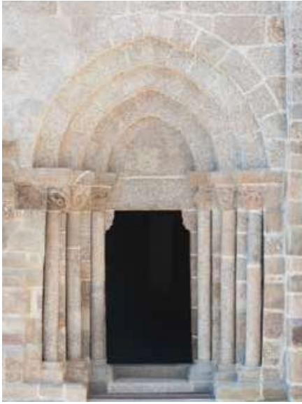
Church. North façade. Nave. Portal.
