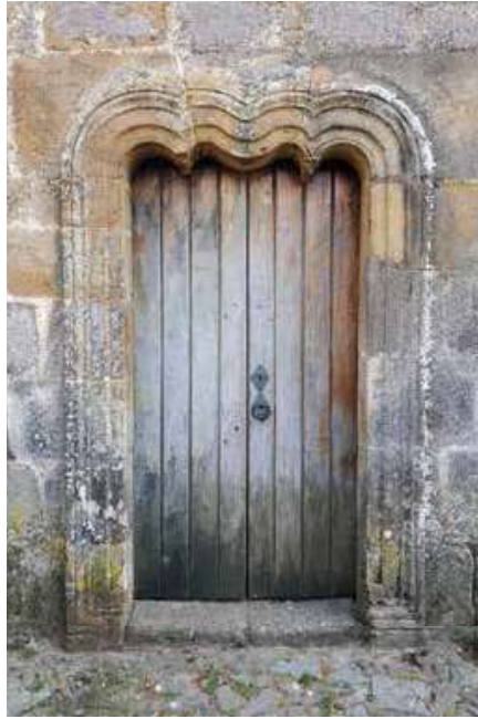
Church, North façade. Nave. Portal.
