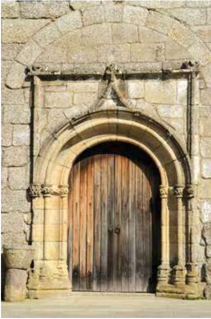
Church, West façade. Portal.
