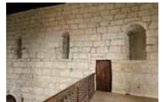
Church. South façade. Nave.
