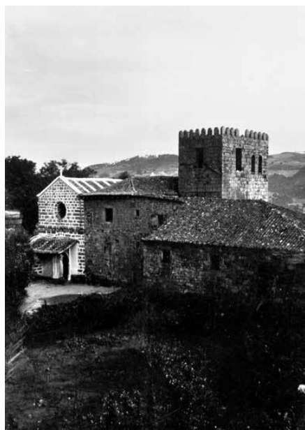
View of the Monastery before the intervention carried out by the DGEMN. Source: Nuno Resende's private collection.
