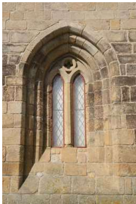
Church. East façade. Mullioned window.
