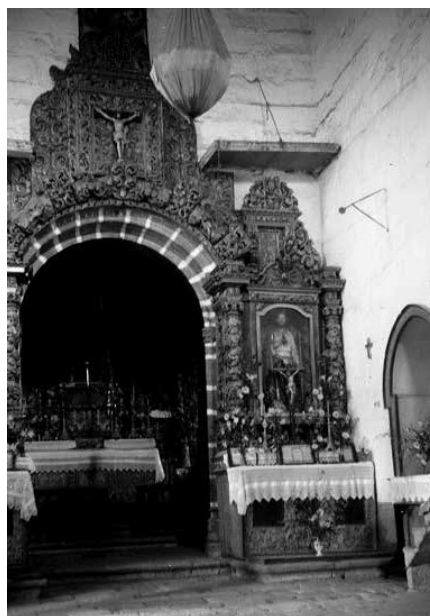
Church. Interior before the intervention carried out by the DGEMN. Source: IHRU archive.
