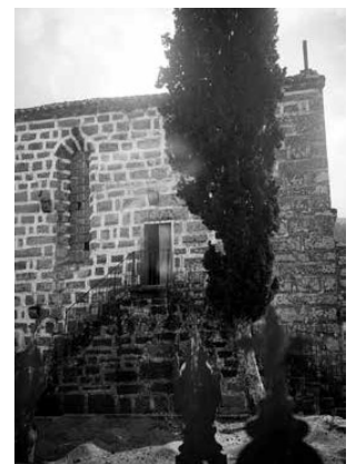
Church. North façade before the intervention carried out by the DGEMN. Source: IHRU archive.
