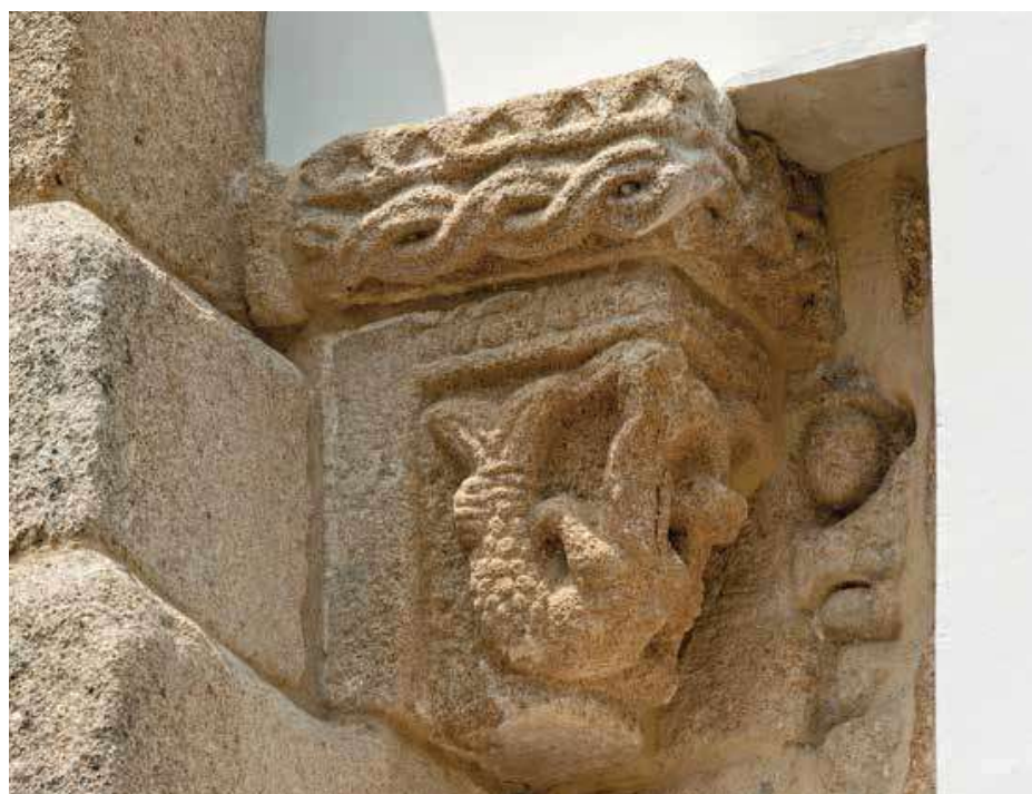
Church, South façade. Chancel. Capital.
