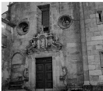
West façade before the intervention carried out in the 1990’s. Source: IHRU archive.
