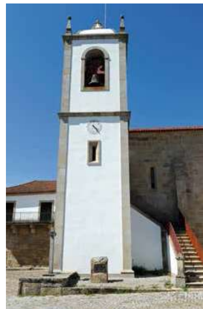
South façade. Bell tower.
