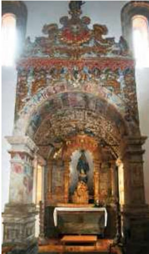
Church. Nave. South wall. Chapel of the Blessed Sacrament.
