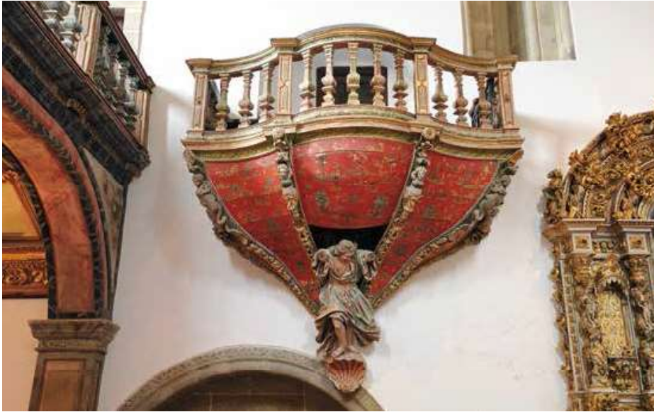
Church. Nave. North wall. Balcony.
