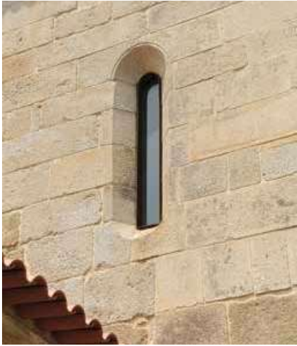
Church. South façade. Nave. Crevice. External view.
