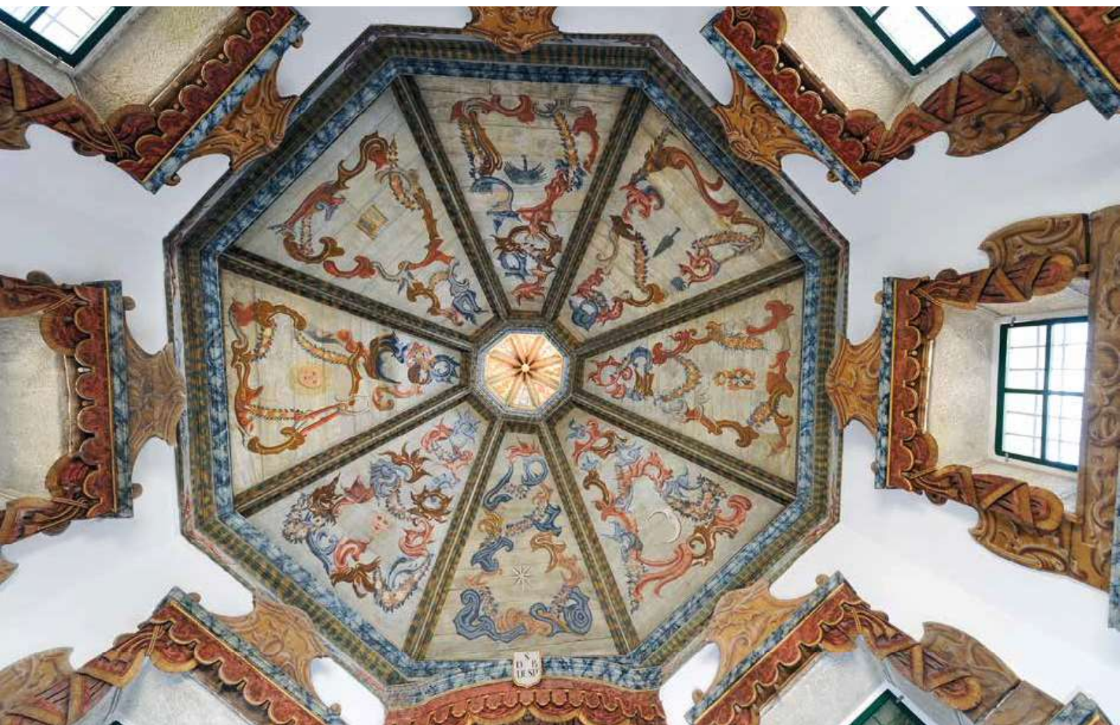
Chapel of the Lord of the Good Delivery. Nave. Roof.
