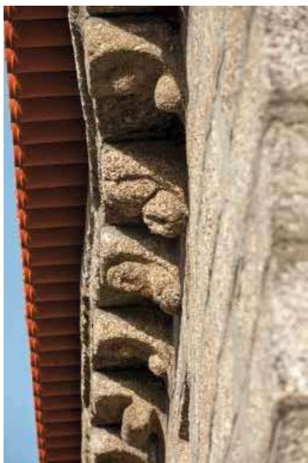
North façade. Nave. Corbels.
