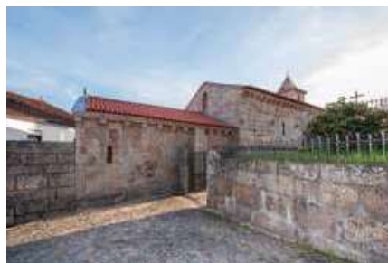
North façade. Chancel.
