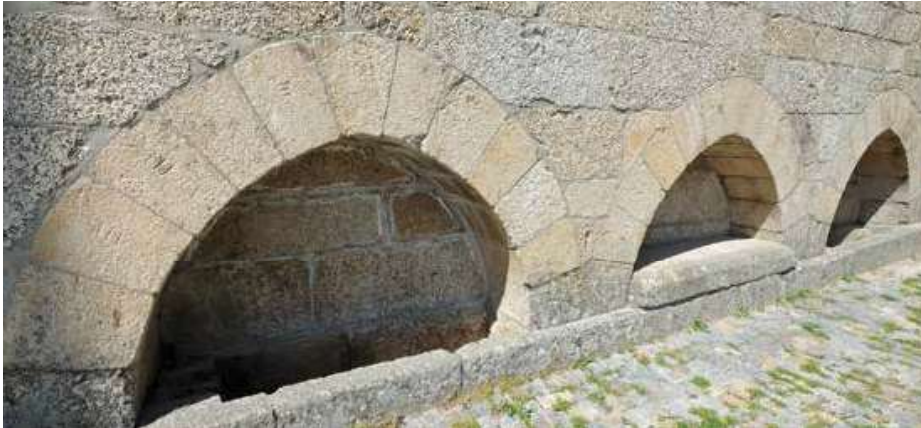
South façade. Nave. Arcosolia.
