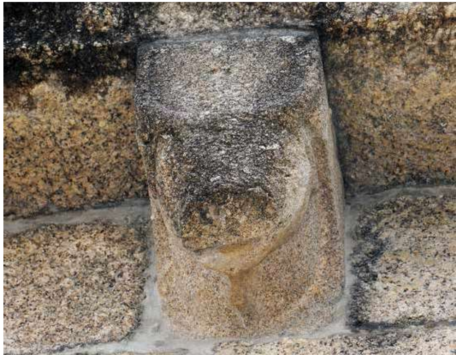
North wall. Nave. Corbel.
