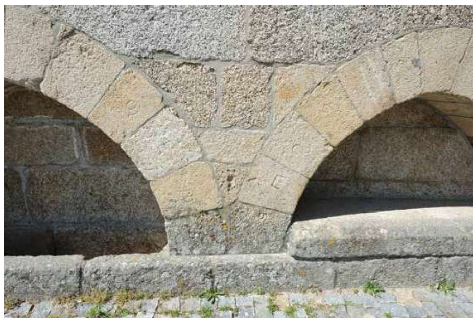
South façade. Nave. Arcosolia. Voussoirs. Initials.
