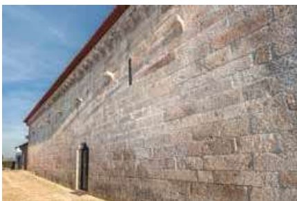
North façade. Nave.
