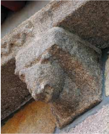
South façade. Nave. Corbel.
