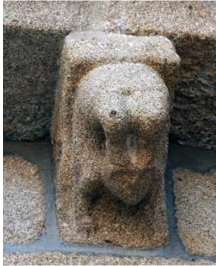
South façade. Nave. Corbel.
