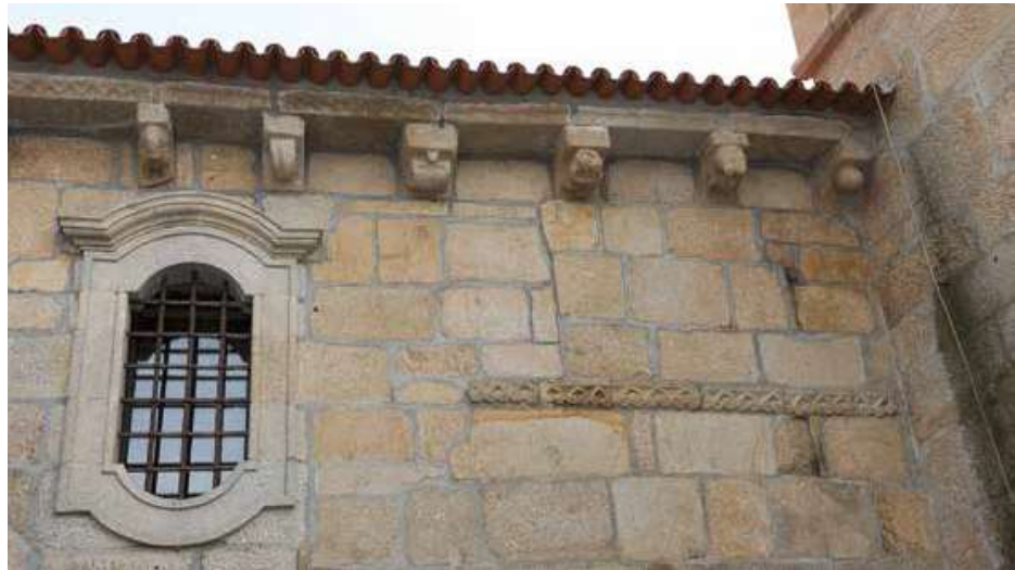
North façade. Nave. Frieze and later works.
