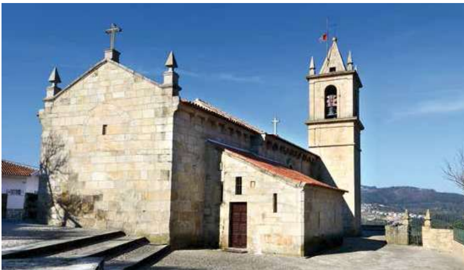
East and north façades.
