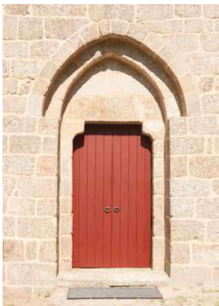
Church of Saint Nicholas. North façade. Nave. Portal.
