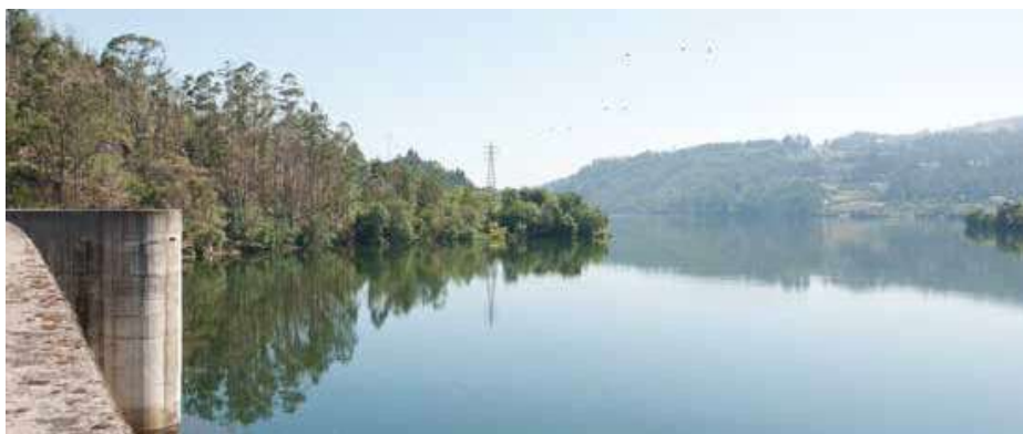
Torrão dam. View of the reservoir.
