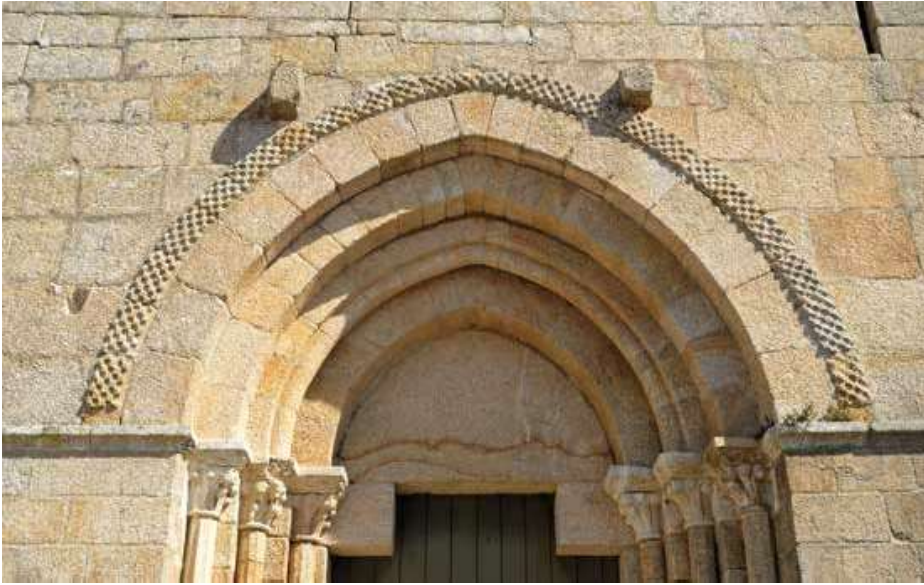
West façade. Portal.
