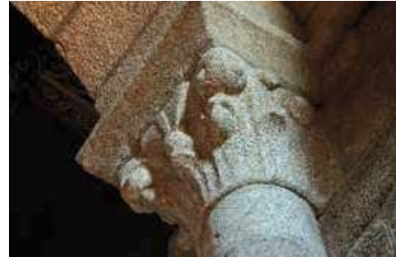
Nave. Capital from the first bay.
