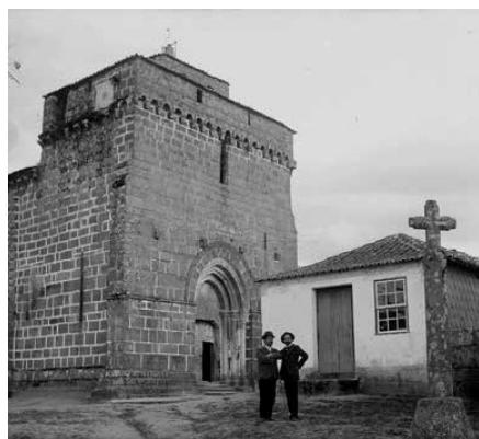
West façade and churchyard before the intervention carried out by the DGEMN. Source: IHRU archive.
