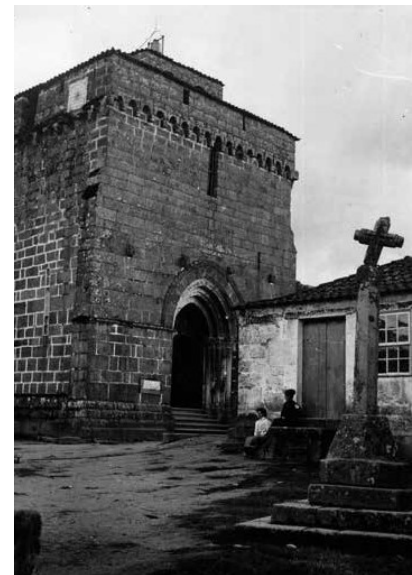
West façade and churchyard before the intervention carried out by the DGEMN. Source: Nuno Resende's private collection.
