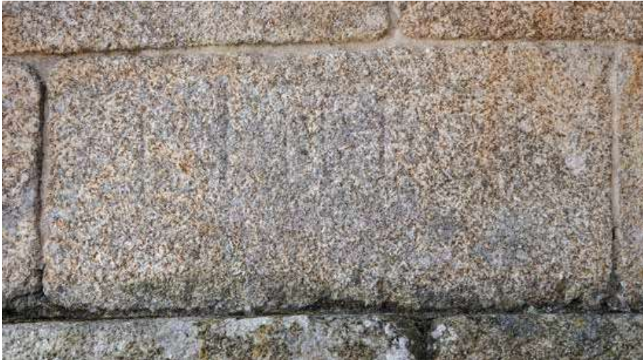
North façade. Chancel. Commemorative inscription marking the Church's construction.
