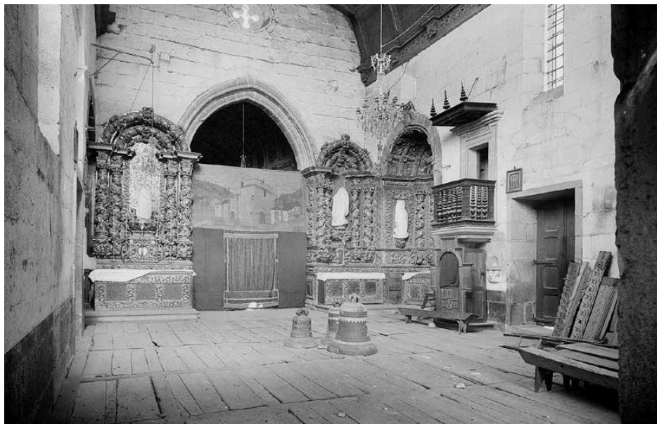
Intervention in the nave (1946). Source: IHRU archive.
