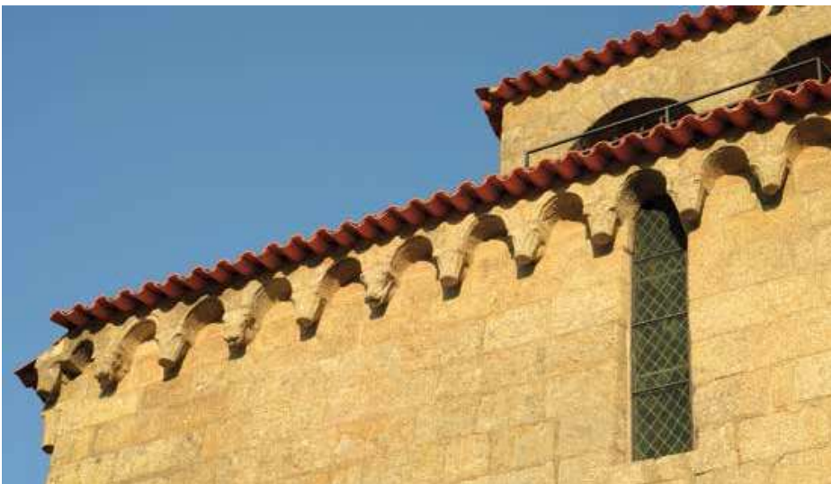
West façade. Corbels.
