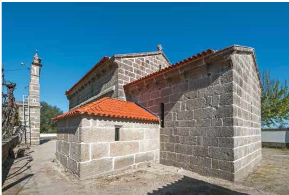
East and south façades.
