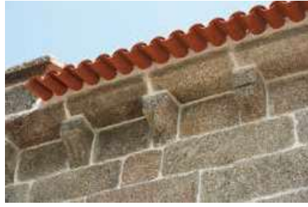
South façade. Chancel. Corbels.
