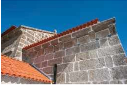
South façade. Chancel. Cornice.
