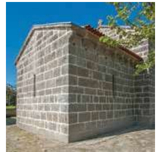
East and north façades. Chancel.
