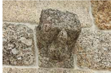
South façade. Nave. Corbel.
