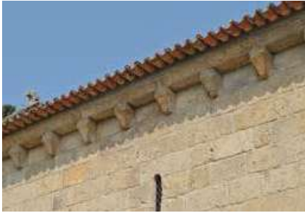
South façade. Nave. Corbels.
