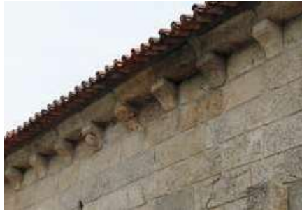
North façade. Nave. Corbels.
