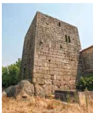
General view before the intervention carried out by the Route of the Romanesque (2014).
