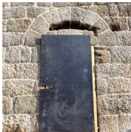
Northeast façade. View from the door during the intervention carried out by the Route of the Romanesque (2014).
