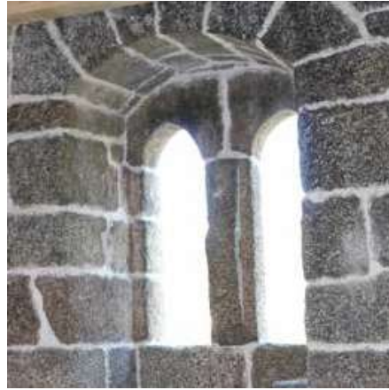
Northeast façade. Upper floor. Detail of the mullioned window. Interior view.
