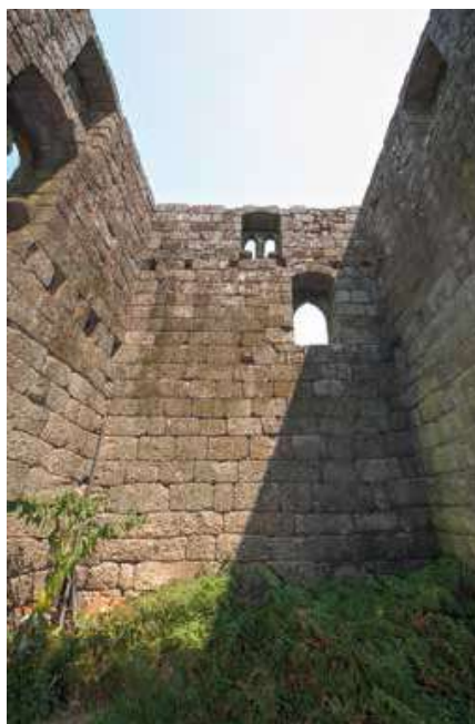
General view of the interior walls before the intervention carried out by the Route of the Romanesque (2014).
