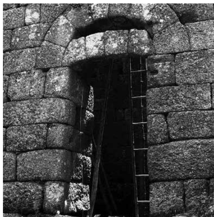
Northeast façade. Door (1951). Source: IHRU archive.
