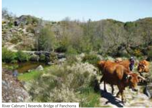
River Cabrum | Resende. Bridge of Panchorra
