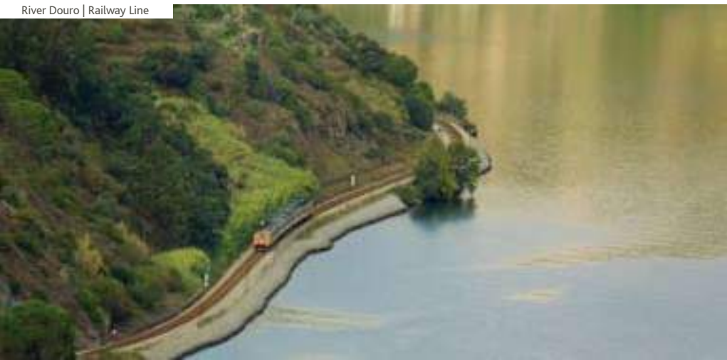
River Douro | Railway Line
