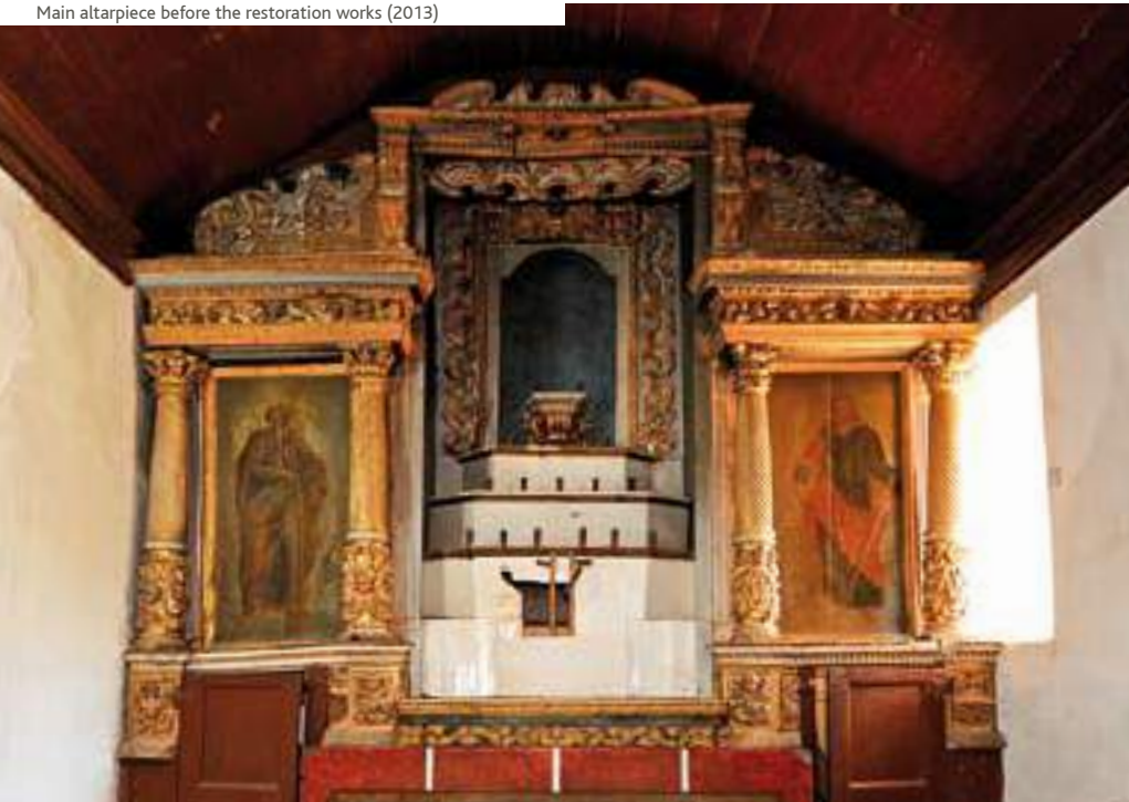
Main altarpiece before the restoration works (2013)
