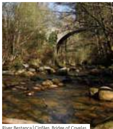
River Bestança | Cinfães. Bridge of Covelas
