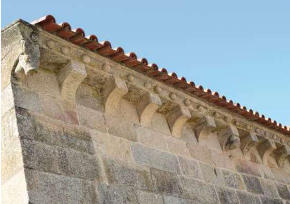
North façade. Chancel. Corbels.
