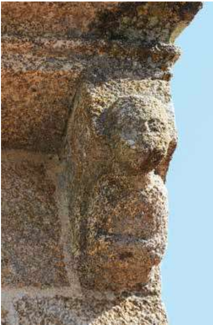
South façade. Nave. Corbel.
