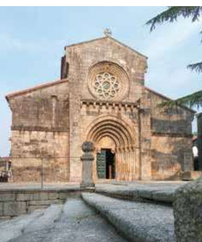
Monastery of Paço de Sousa (Penafiel). West façade.
