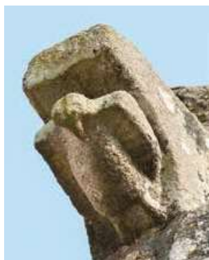
North façade. Corbel.
