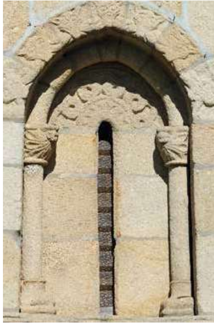
South façade. Crevice.
