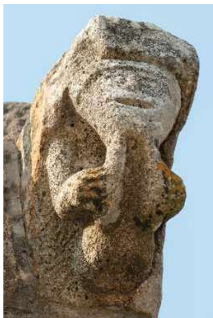
South façade. Corbel.
