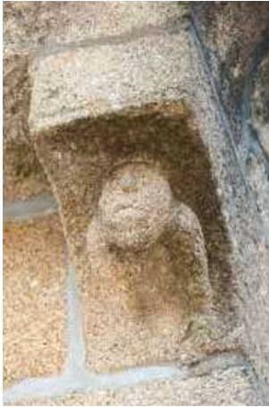
South façade. Corbel.
