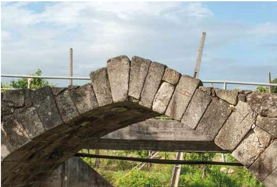
Downstream view. Arch top.
