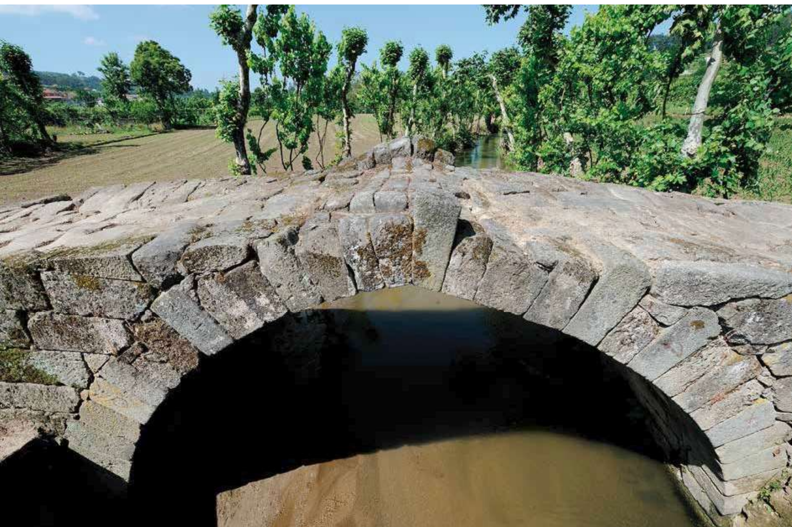
Upstream view. Arch and platform.
