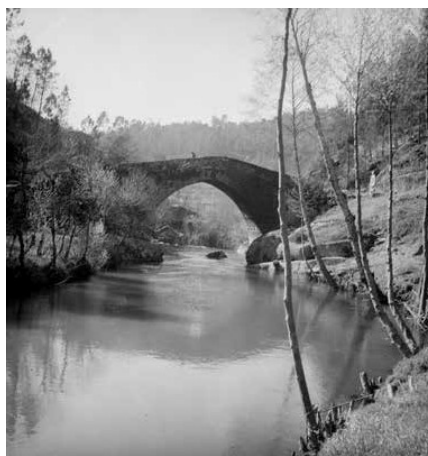
Upstream view (1977). Source: IHRU archive.
