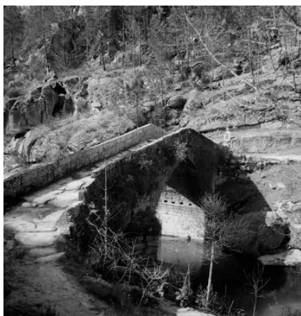
Upstream view (1977). Source: IHRU archive.
