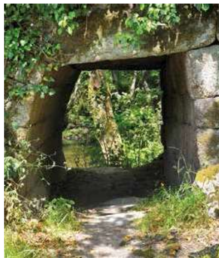
Detail of the drainage channel.
