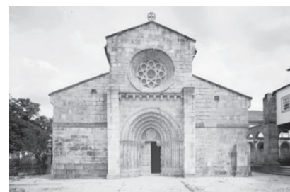
32. West façade after the intervention of the DGEMN.
