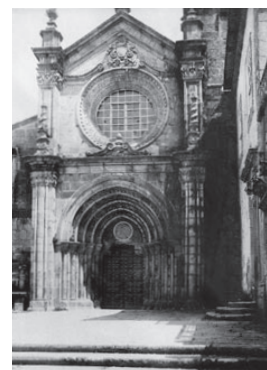
27. West façade before the intervention of the DGEMN.
