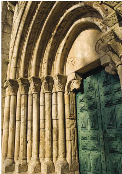
4. West portal. The prismatic columns, the motives used in the capitals and the bulbed bases characterize the typical sculpture from the Basins of the Sousa and Lower Tâmega.
