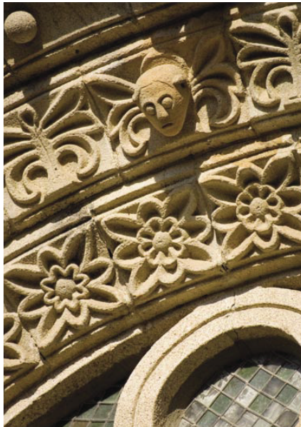
19. West façade's rosette. Frame.
