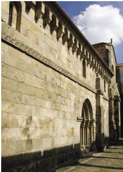
3. Church's South façade. The cloister and monastic ensemble were built on the church's South side.
