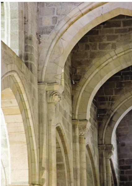
12. The use of diaphragm arches on the naves' roofing is a solution that is reminiscent of the partitioning of the space in Peninsular Pre-Romanesque churches.
