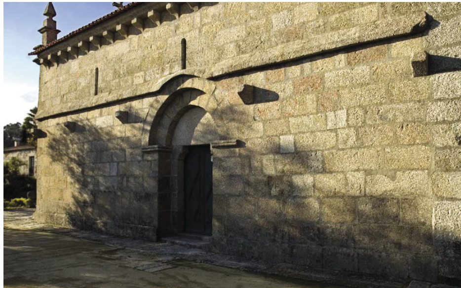
3. South side façade. The drip course and the corbels testify to the existence of a porch.
