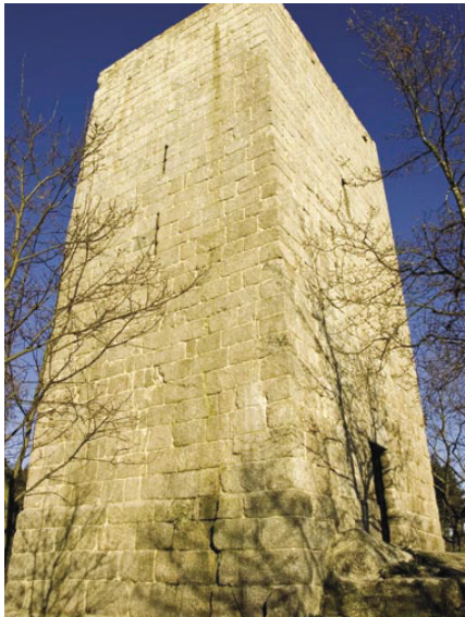
2. The Tower's walls are laid directly over the granite rock.
