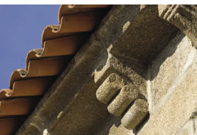
5. South façade . Corbels.
