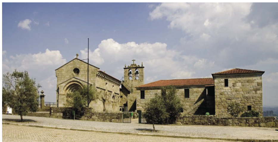
1. The church of Saint Vincent of Sousa is a very well designed building with high quality construction.
