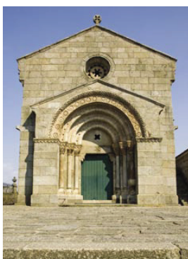
4. West façade. The portal is inserted in a pentagonal structure stemming from the façade, a usual solution in this region, as the church portals of Saint Mary of Airães and of the Savior of Unhão, both in the municipality of Felgueiras, demonstrate.
