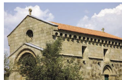
10. West and South façades. The South façade is topped by a cornice over small arches, a common solution to Saint Mary of Airães (Felgueiras) and Saint Peter of Ferreira (Paços de Ferreira).
