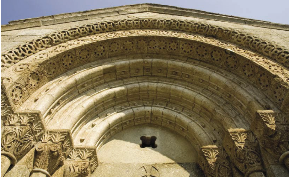
9. West portal. The parallels with reminiscent elements from the See of Porto's West portal.
