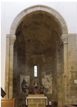
7. South apsidiole. The transepts with apse and step apsidioles, of semi-circular design, are common in the programs for churches bearing three naves in the region between Douro and Minho rivers.
