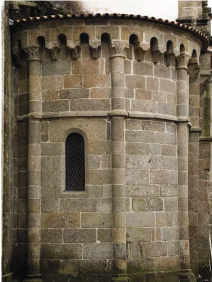
8. Apsiole. The arch cornice set in corbels finds parallels in the churches of the Monasteries of Saint Peter of Ferreira and the Savior of Paço de Sousa, among other Romanesque temples of the Sousa Valley.
