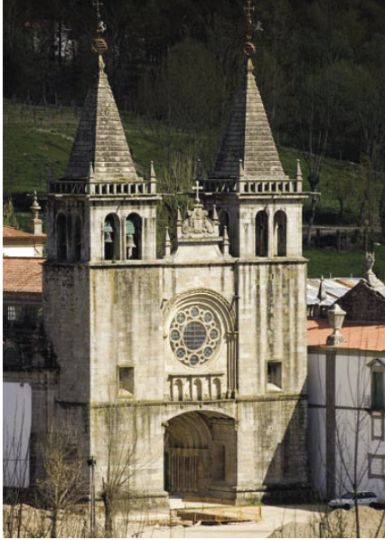
5. In spite of the Modern period's restoration, the church's structure corresponds to the Romanesque construction, with the exception of the main chapel, erected in 1770.
